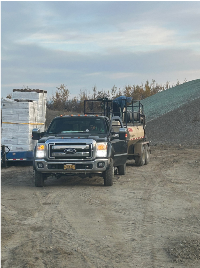
Hydroseeding completed on Cell 2 stockpiles as required by Department of Environmental Conservation September 29, 2023
