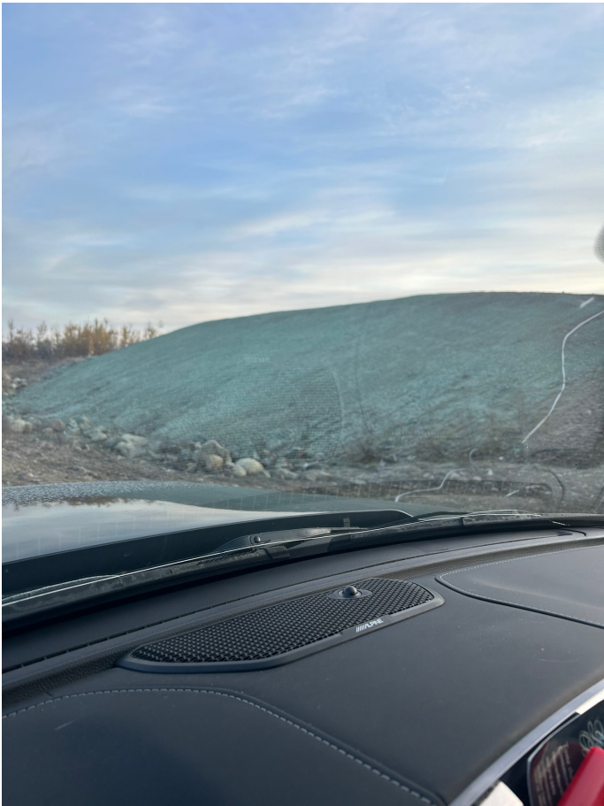
Hydroseeding completed on Cell 2 stockpiles as required by Department of Environmental Conservation September 29, 2023
